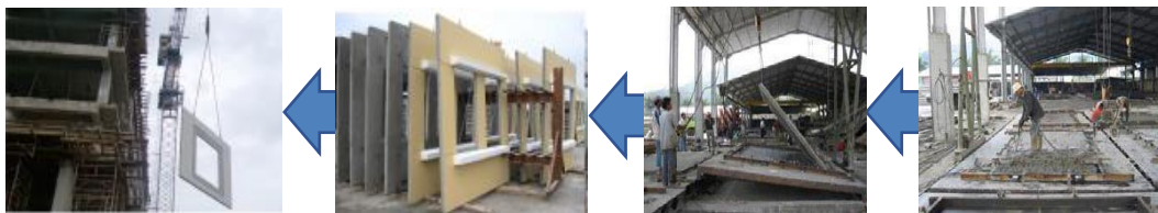
Figure 3. Curtain Wall Facade
