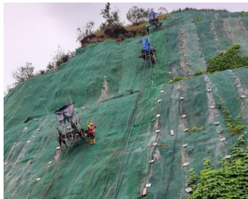
Picture 6 Slope Treatment Works uses Hanging Platform
