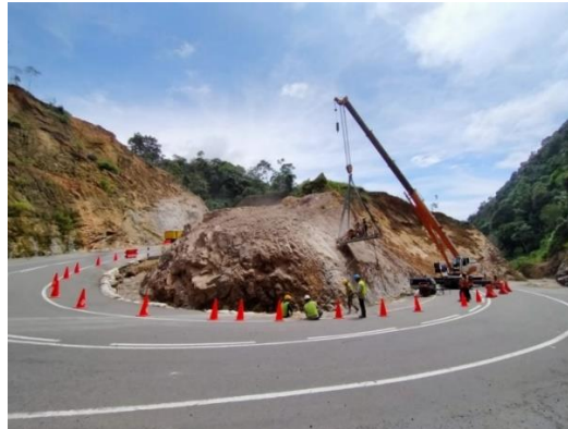
Picture 1 Anchor installation using Transport Equipment Manlift Source: Documentation Project, 2020
