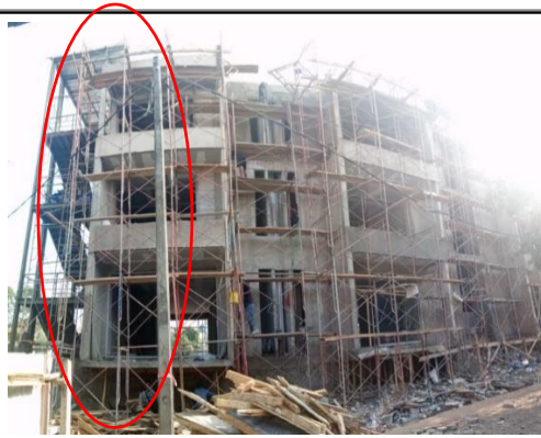
Picture 7 frame Scaffolding
