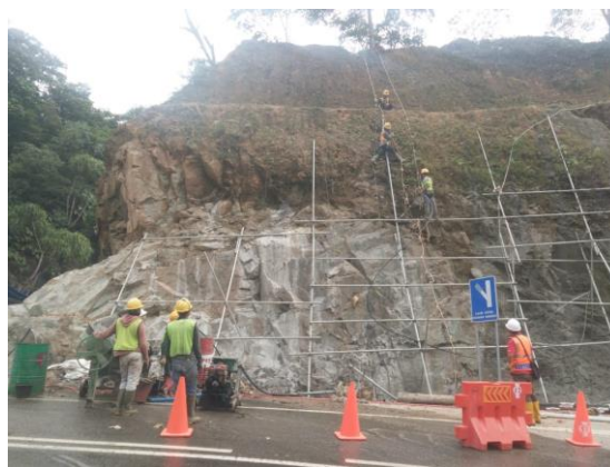
Picture 2 Anchor installation using pipe Scaffolding Source: Documentation Project, 2020
