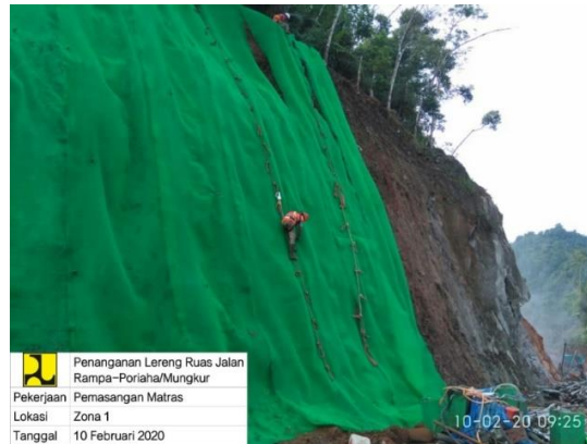
Picture 3 Installation Work Wire Mesh Source: Documentation Project, 2020
